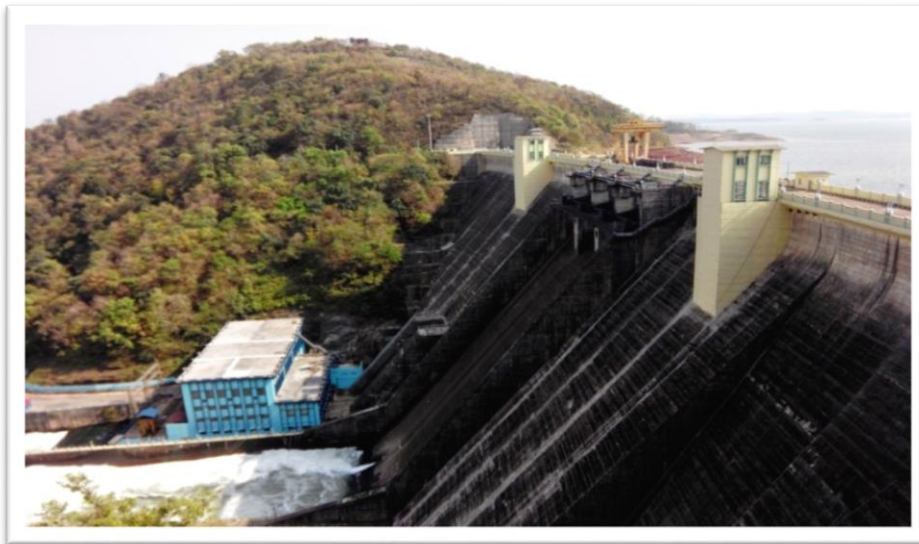
Supa dam and Power Station, Uttar Kannada
